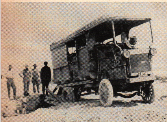
Three miles outside Kenton, Utah, farmers gathered to watch crew repair wooden bridge which collapsed.
